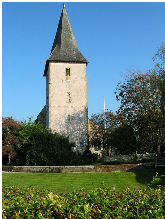
Bosham Church: the lower three storeys of the tower are Saxon, the top storey Norman
