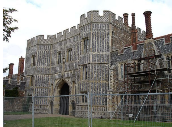
Gatehouse of the former St Osyth's Priory (later abbey), St Osyth, Essex
